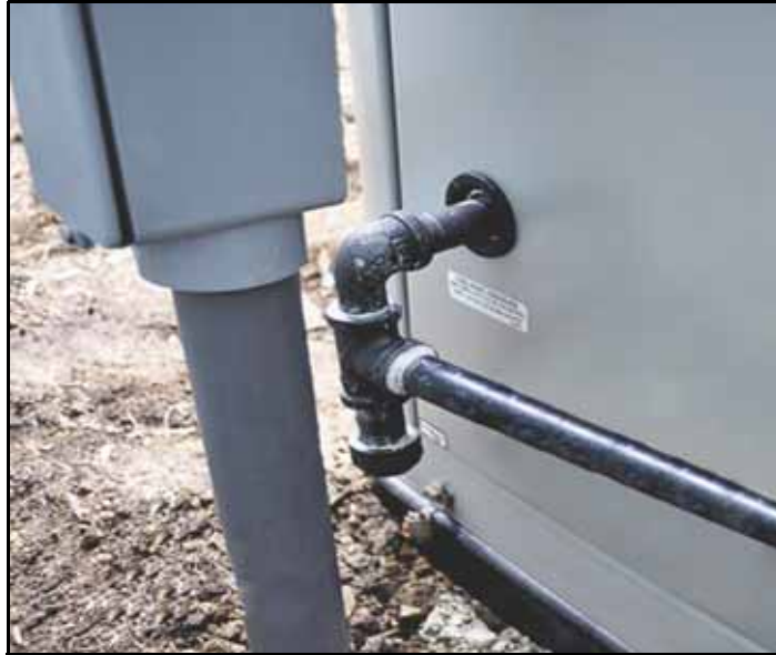
Figure 5-3. Sediment Trap (typical)
